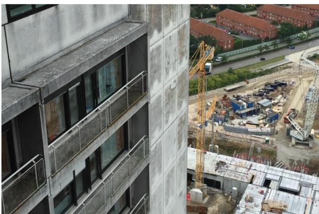
**Fig. 1:** *The concrete façade inspection in Herlev Hospital was performed using ropes and lifts.*
